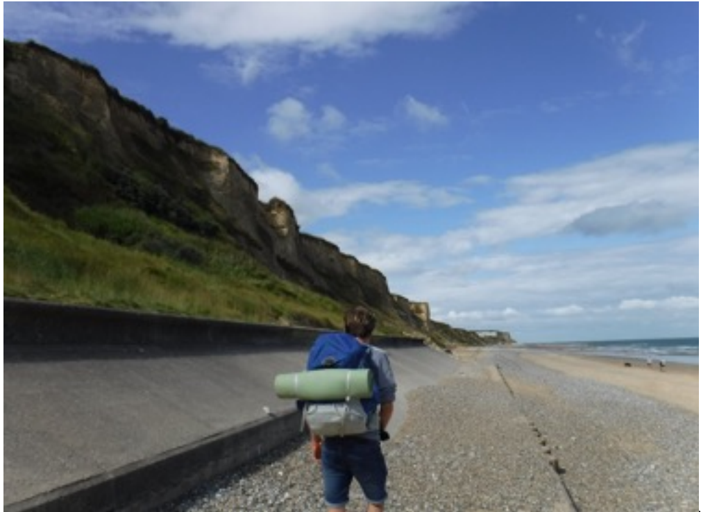
Cliff and Sea Wall, East Runton
