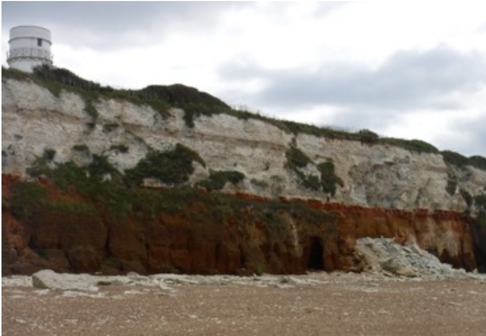
Sheer cliff erosion with Caves, Hunstanton
