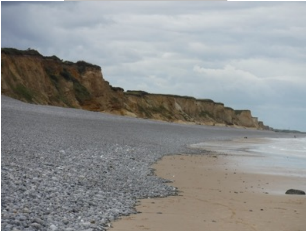
Cliff erosion, Weybourne
