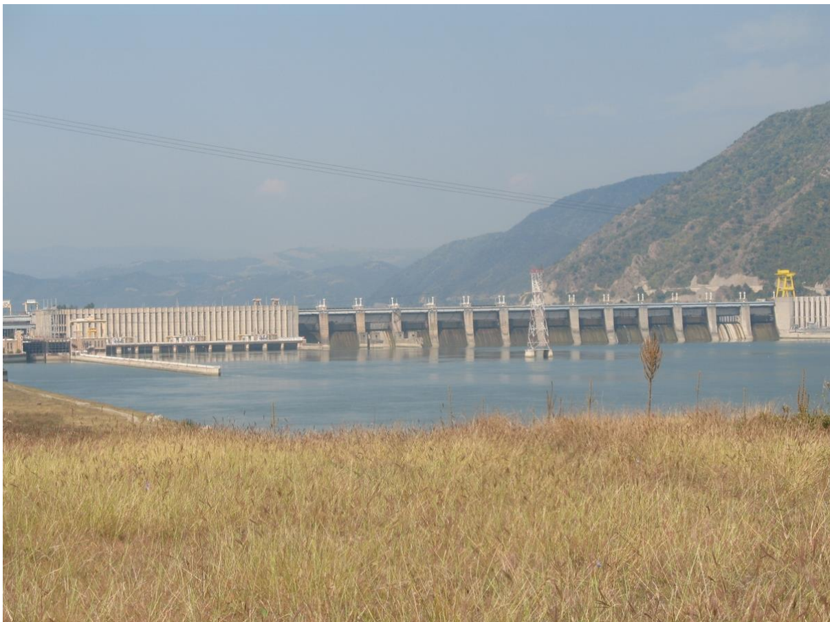
Figure 16: The Iron Gates Hydroelectric Station
