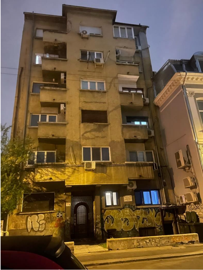
Figure 32: Example of an apartment building in Bucharest
