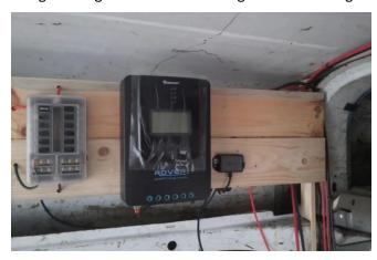
seat for the power to go into. The power from the solar panel would travel through a converter and into the battery. The energy stored in the battery would then have to get split into 2 types; DC, which would run to the fridge, water pump and air vent; and AC which goes to the lights and sockets.
