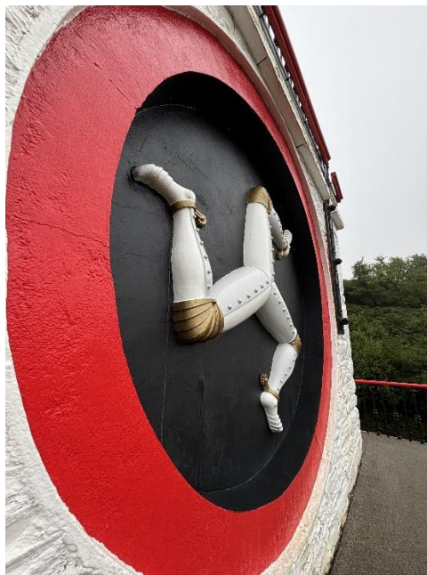
Figure 48: The Triskellion on the front of the wheel. When the symbol was being cast, the people doing it forgot to reverse the image so the Three Legs of Man on the wheel are backwards.
